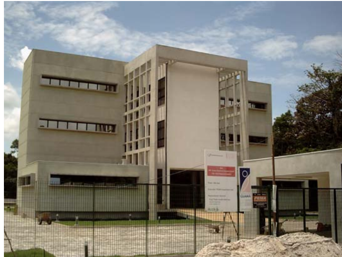
Figure 6. INPE office complex.
